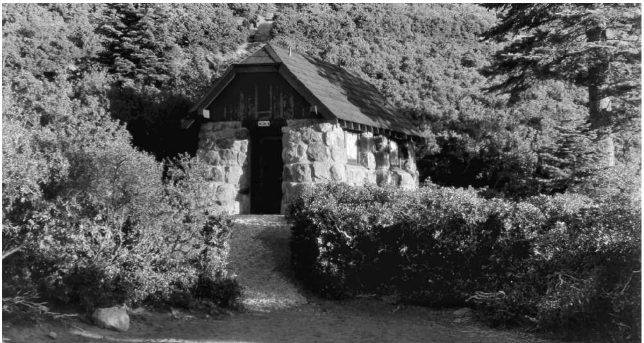
TOP LEFT Comfort station at the stables (2004) GH MIDDLE LEFT Small building at the stables (2004) GH TOP RIGHT Small bathhouse plan and section BOTTOM Comfort station at Union Point (1932) YRL-RA
