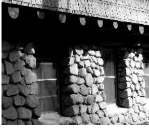
Exterior wall of Administration Building, Yosemite Village (2004) GH
