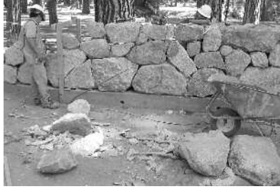
Stone wall under construction at Lower Yosemite Fall area (2004) RF
