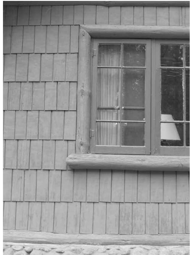
Exterior wall detail from historic wood cabin, Curry Village (2004) RF
