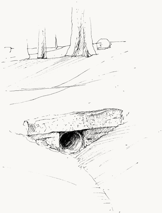
TOP Footbridge BOTTOM Culvert
