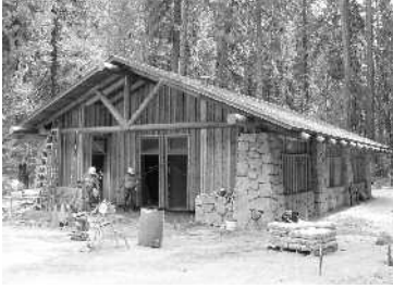
Lower Yosemite Fall comfort station under construction (2004) RF
