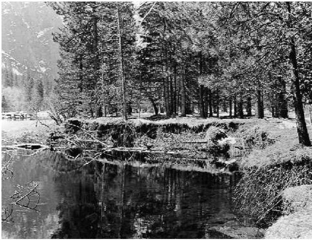
Erosion of river bank near Yosemite Lodge (1929) YRL
