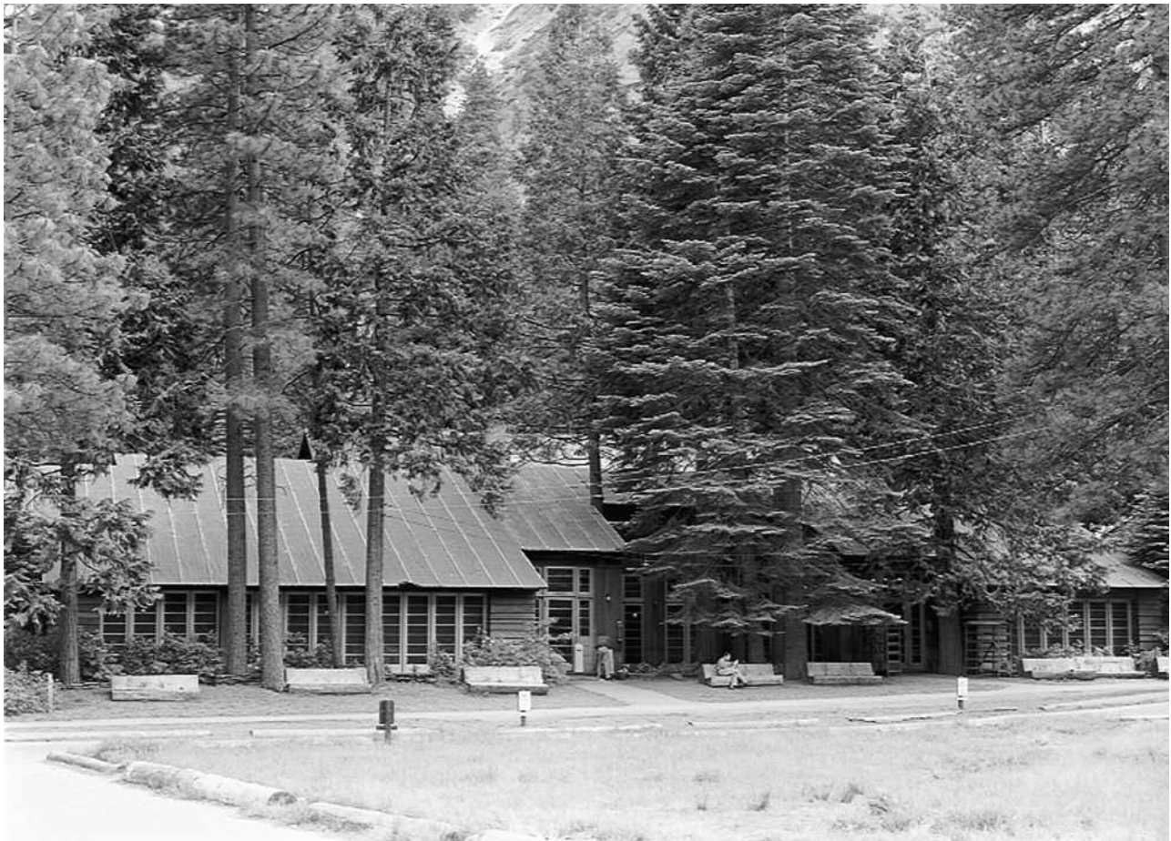
TOP LEFT Mountain Shop window detail TOP RIGHT Mountain Shop bay window BOTTOM Early view of Camp Curry cafeteria (now the Mountain Shop). The building was notched to accommodate the large conifers. Conifers have since been replaced with a deck. (date unknown) YRL
