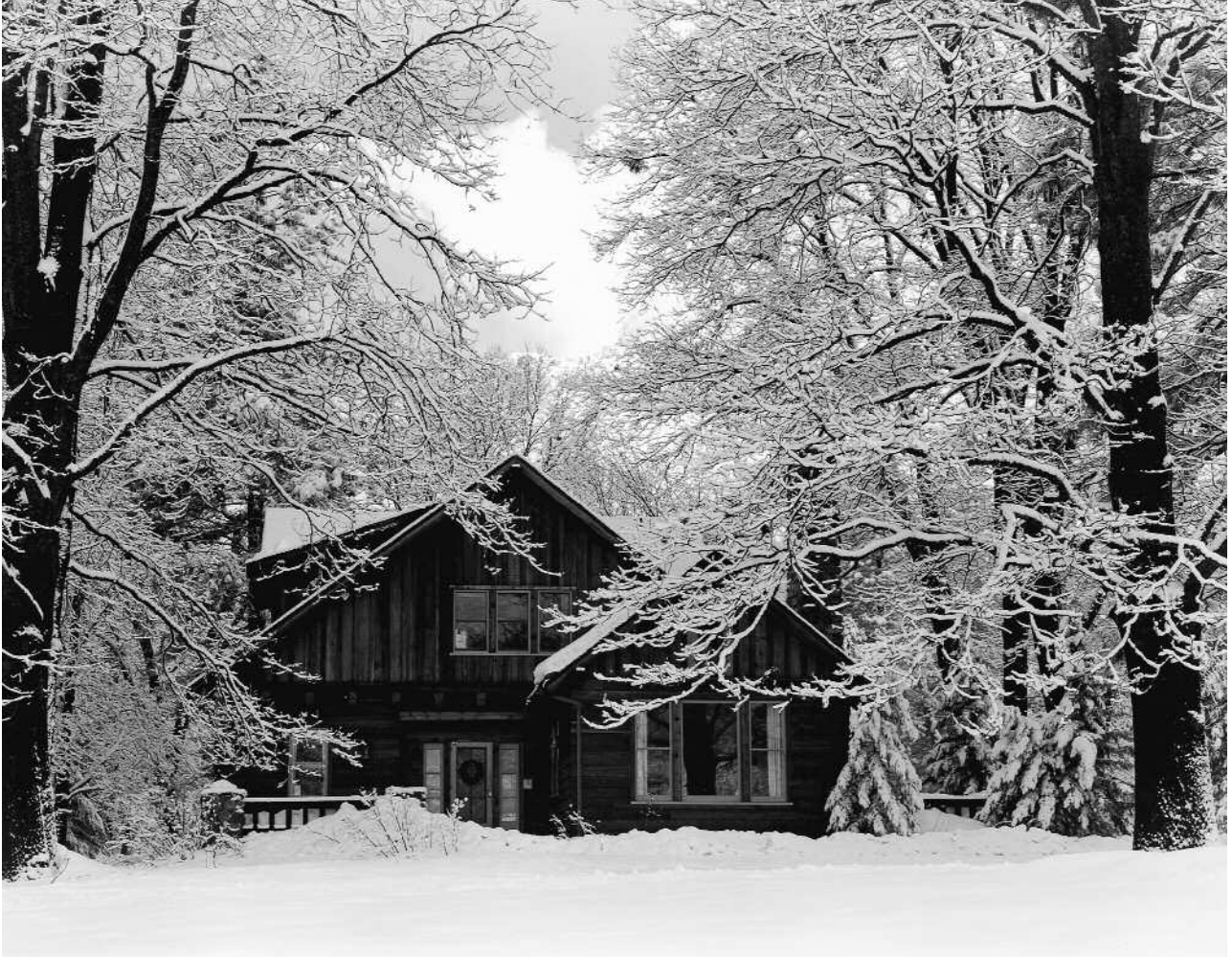
Superintendent's House (Residence I), Yosemite Village (1942) YRL-RA
