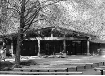
Porch entry to Mountain Room Restaurant linking cafeterias and restrooms (2004) GH
